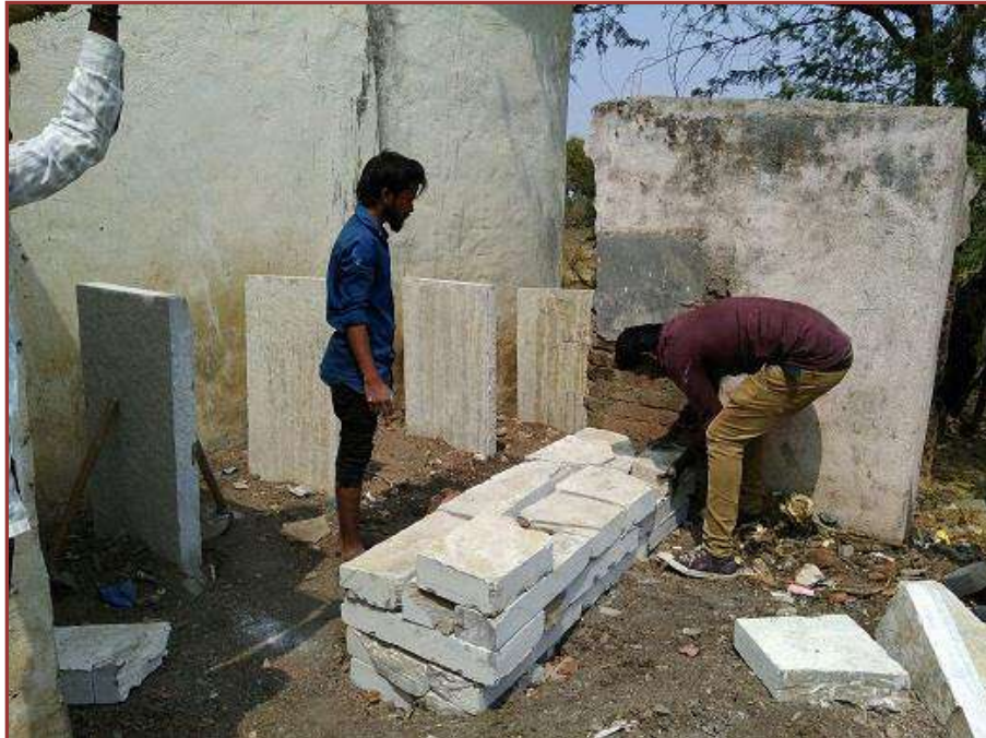
N.S.S Volunteers constructing toilets for students in Govt. School, Tonasanahalli(s)
